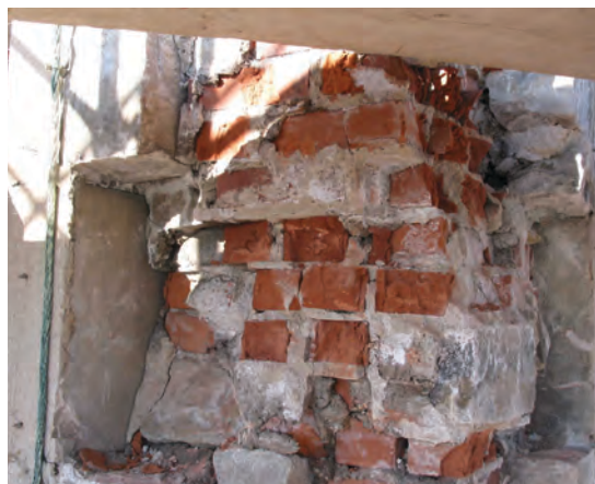
Fig. 2. Brick failure at Saint Paul's Church, Cranston, Rhode Island, 2002. This mass brick masonry was set with a portland-cement mortar that has failed due to decades of water infiltration and freezing and thawing. It is an example of the type of non-sacrificial global assembly failure that occurs with more modern, higher-strength mortar binder materials.
