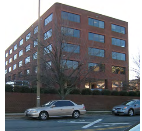
Existing Pipefitters Union Building
