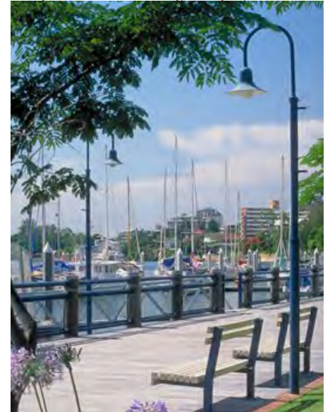
Design details on walkway, Beaufort, NC
