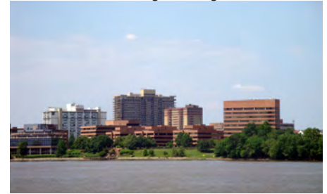
Looking from the water past Tide Lock Park (Crowne Plaza showing in background - left)
