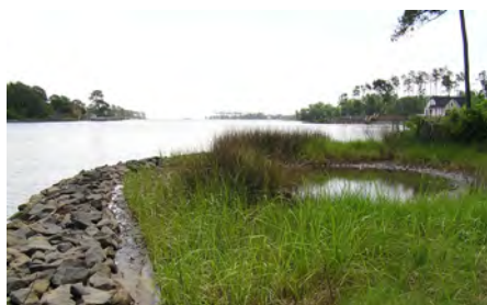
Structural Revetment for Shoreline Naturalization (Center for Coastal Resources Management, Virginia Institute of Marina Science)
