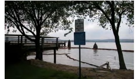
Oronoco Outfall at the foot of Oronoco St.
