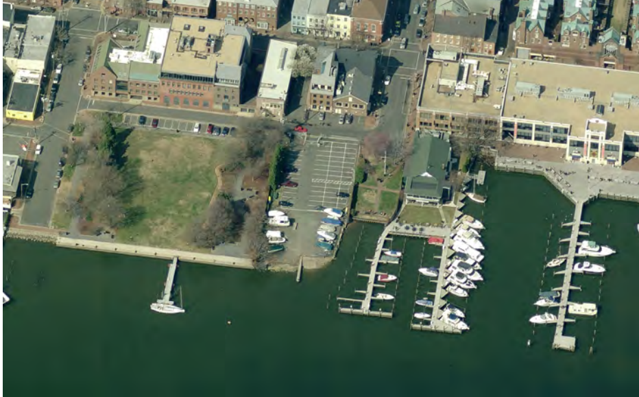
Aerial view of existing condition at the foot of King Street
