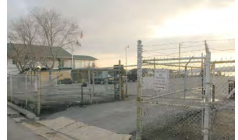
Existing ODBC Parking Lot
