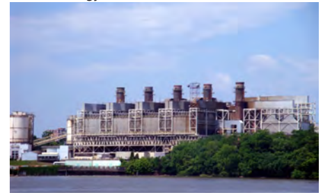
GenOn Energy Power Plant
